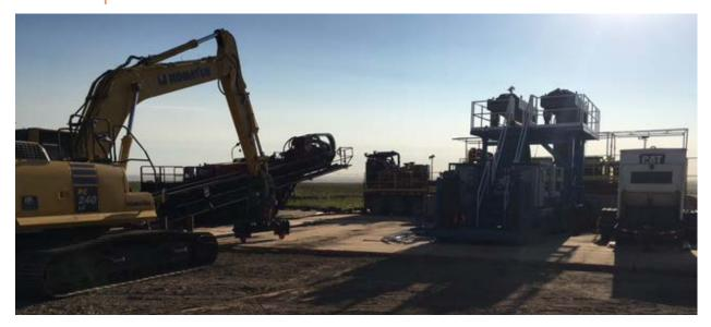
Water testing and water monitoring is taking place at this location, every 100m the pipeline crew have monitors downstream. This way they if there was to be an incident where drilling mud is released into the canal the crews would know right away and be able to respond. Water samples are collected every few hours and turbidity levels are documented.
